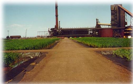
After trials, a large scale (2 ha) trial system was constructed and commissioned in 1997. This involved the adaptation of the plants and biological life within the system to pollutants in the wastewater.
