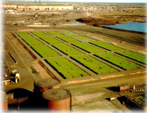
The Whyalla steelworks is located approximately 400 km North of Adelaide, Australia. In Australia, reed beds have been used for storm-water run-off and sewage treatment, but little was known about applications to steelworks wastewater treatment.
