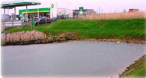
The BP development at Raunds is believed to be the most environmentally friendly service station in the UK! Oceans-ESU Ltd designed a reed bed system that treats all the foul drainage and hydrocarbon-contaminated surface run-off, while ensuring safe operation of the facilities in terms of odour and contamination risk. The treated water is discharged into a stream.
